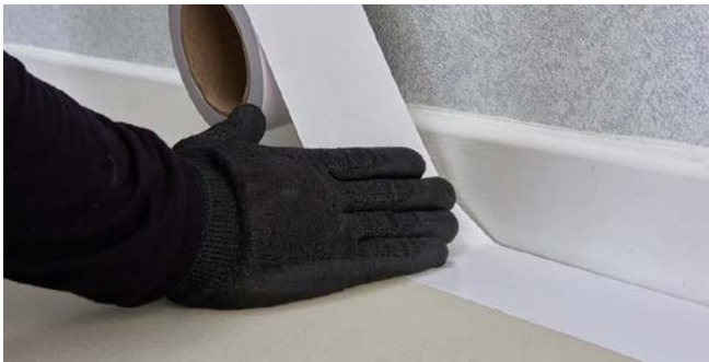
Figure 12 Use double sided Polyflor recommended tape
