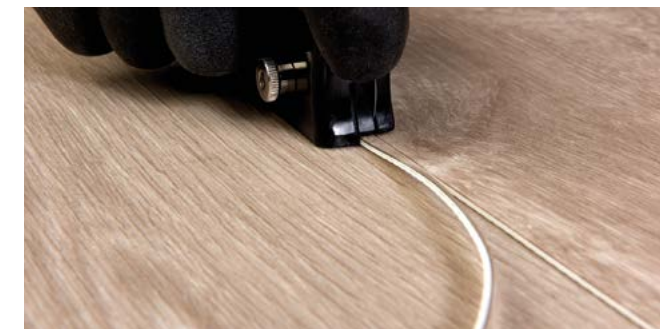
Figure 5 Cutting in the seams
