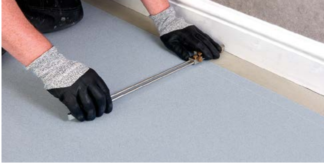
Figure 11 Scribing the wall profile
