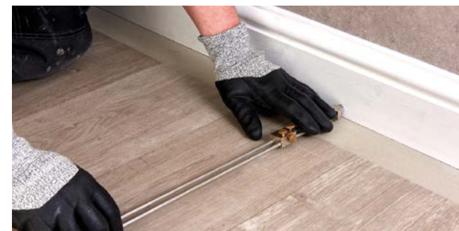
Figure 2 Scribing the wall profile
